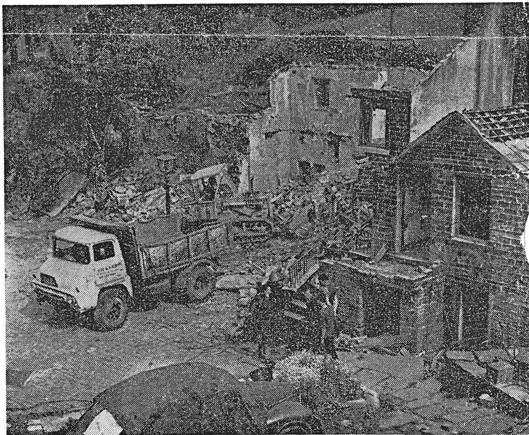
The picture shows work in progress on clearing the site.
